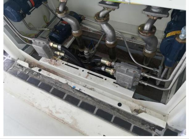
渗漏检测仪、液位监控仪
